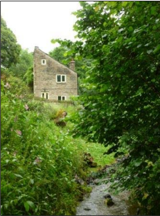
Brookside viewed from Mill Brook
