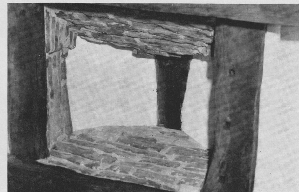
The portion of the medieval "smoke-hole" in the roof, which has been preserved by the present owners
